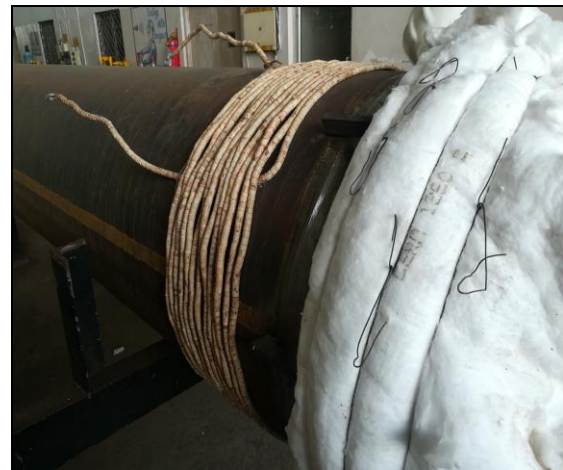
Fig. 4: Post Weld Heat Treatment Process.
