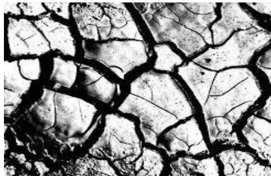
Fig. 1: Cracks in Expansive Soil when Soil is Dry.
