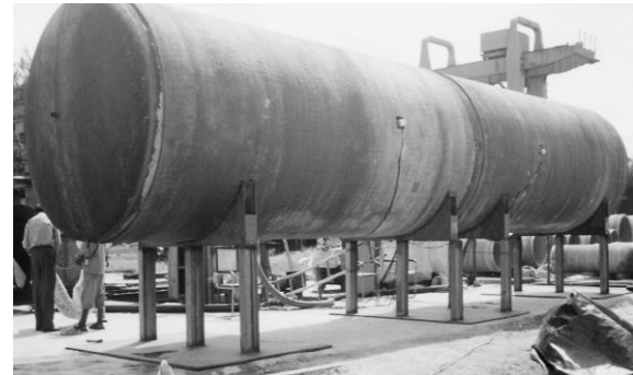
Fig. 2: Prototype Hydrostatic Test Setup of Lined Steel Pipes.
