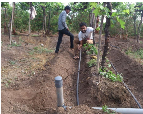
Fig. 1: Installation of SDI.
