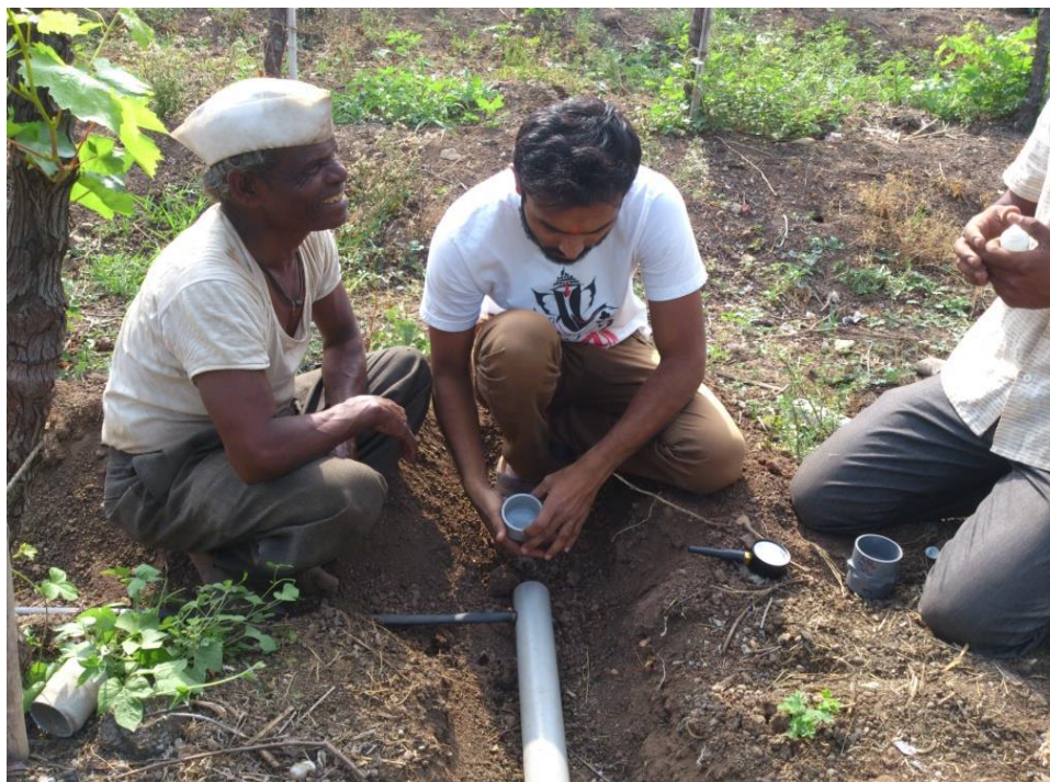
Fig. 5: Making of Flushing End.
