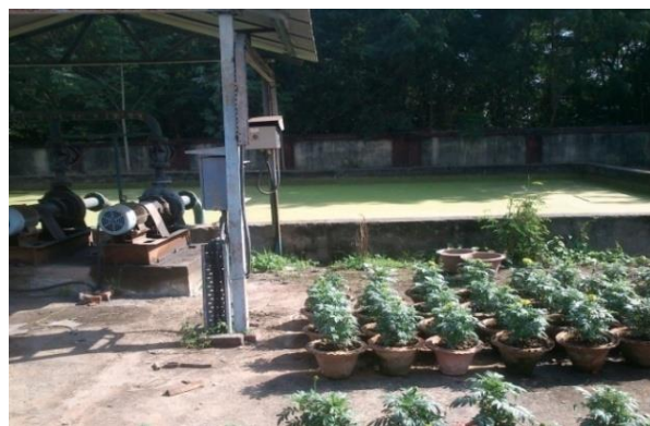
Fig. 9: Storage Tank and Reuse of Wastewater after Treatment for Gardening Purpose.
