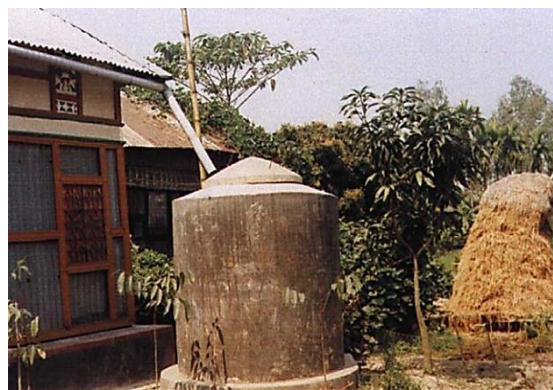
Fig. 7: Rain Water Harvesting System.
